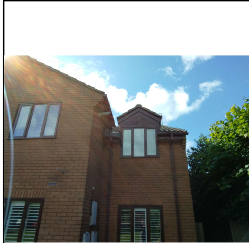
Guttering (Gutters and Fascia)
