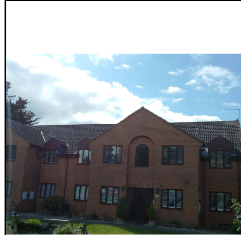
Roofing (Tiles and Cladding)
